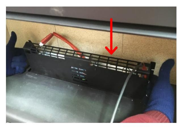
Ensure there is NO Gap at the top between the fan and the heater.
