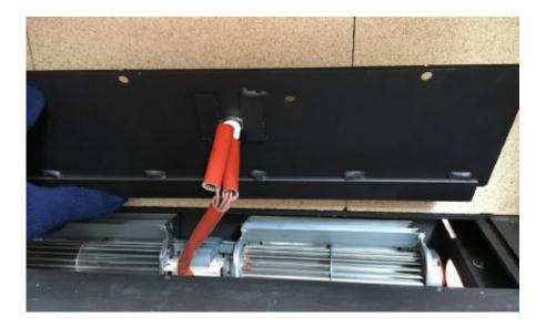
When inserting, ensure that the thermostat cabling is fastened in position <u>so it cannot</u> <u>move and rub or get caught in the fan blades</u>. Besides being noisy, this could damage the cables, the blades and the fan.
